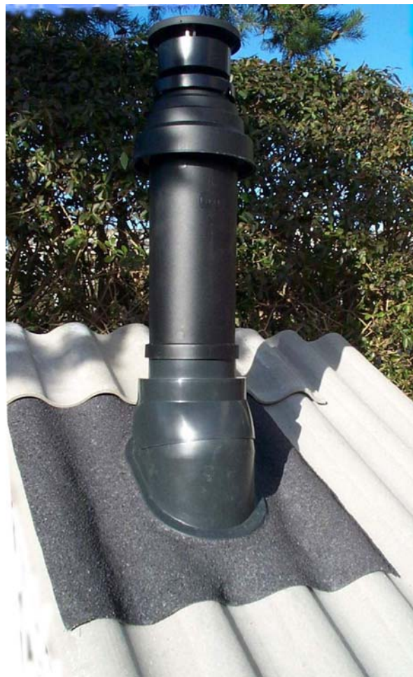
Bosch adjustable roof tile fitted with Perform
